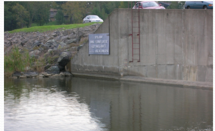
RETAINING ("WING") WALLS
