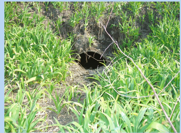
Culvert Diversion – Song Lake
