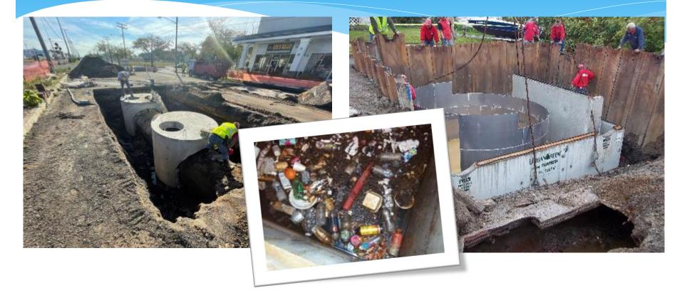
Due to limited open space use both large and small subsurface MTDs to treat stormwater runoff... effective means of controlling floatables, sediment, particulate pollutants and nutrients... inspected quarterly and cleaned out
